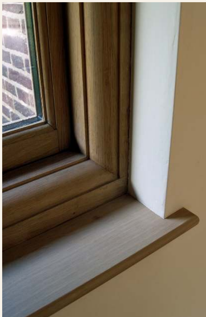
OAK WINDOW SILL & REVEAL DETAIL
