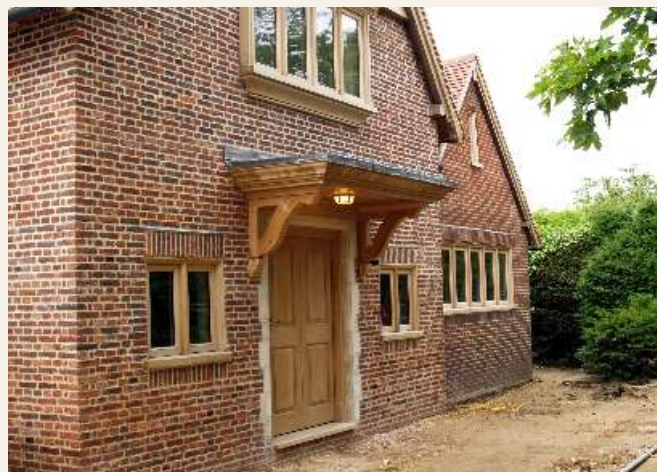
OAK ENTRANCE DOOR & CARVED CANOPY
