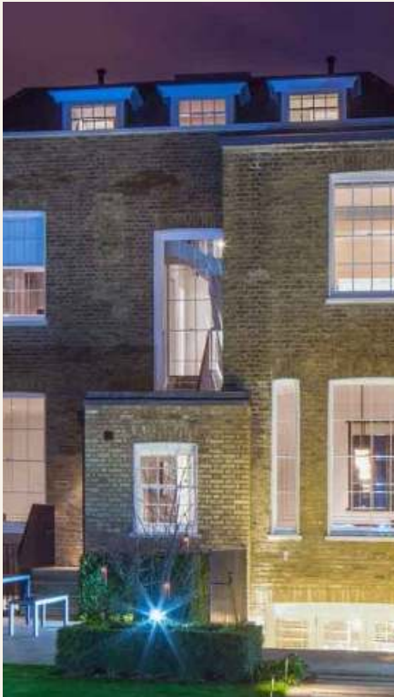
BOX SASH WINDOWS, PAINTED
