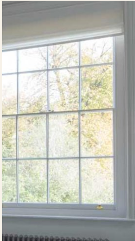
BOX SASH WINDOW DETAIL
