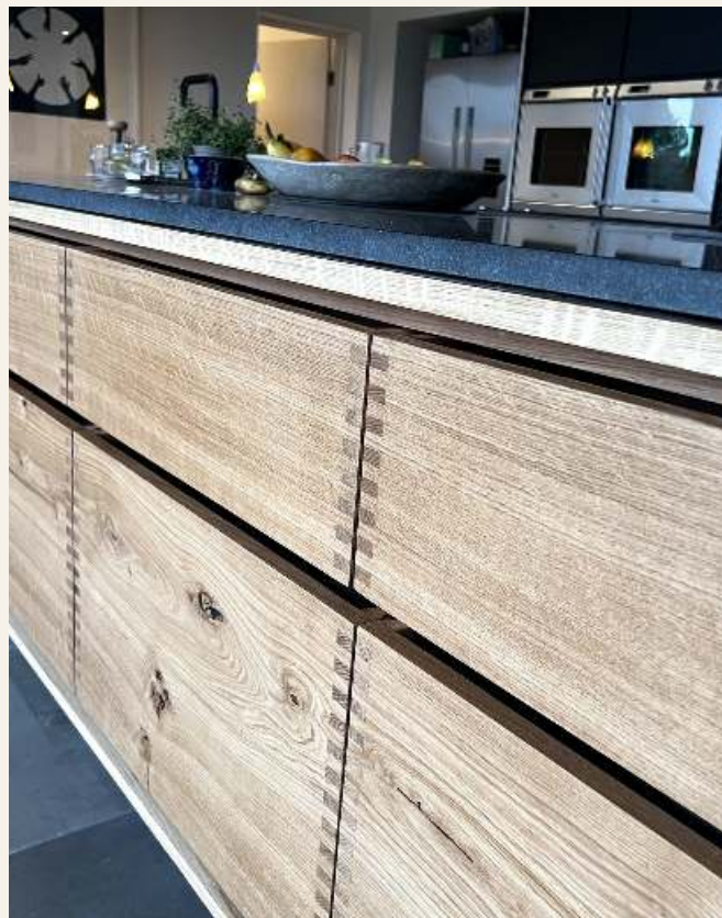
OAK CABINET RUN, DOVETAILED FRONTS
