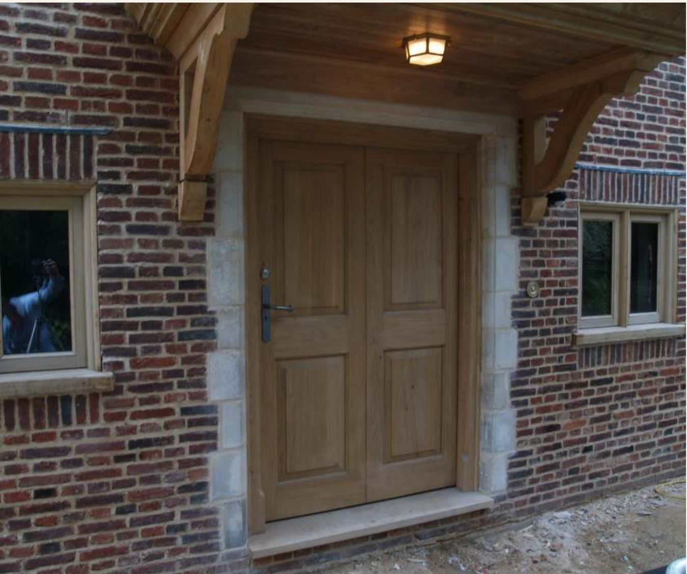
FRONT DOOR WITH OAK CANOPY PORCH
